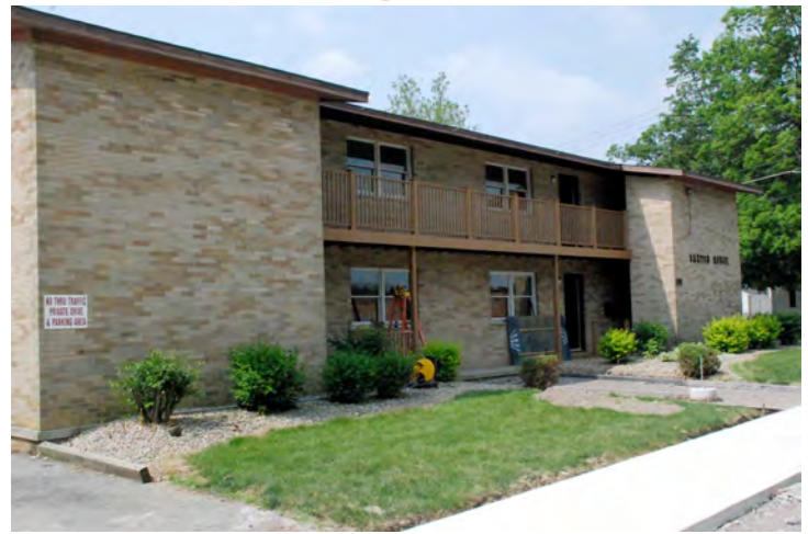
Oiler Pointe, UF's newest housing option for students, is being renovated for fall. The apartments offer a substance-free housing option.
